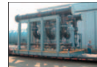
Filtration unit for injection water with three BOLL automatic filters type 6.18, DN 400
